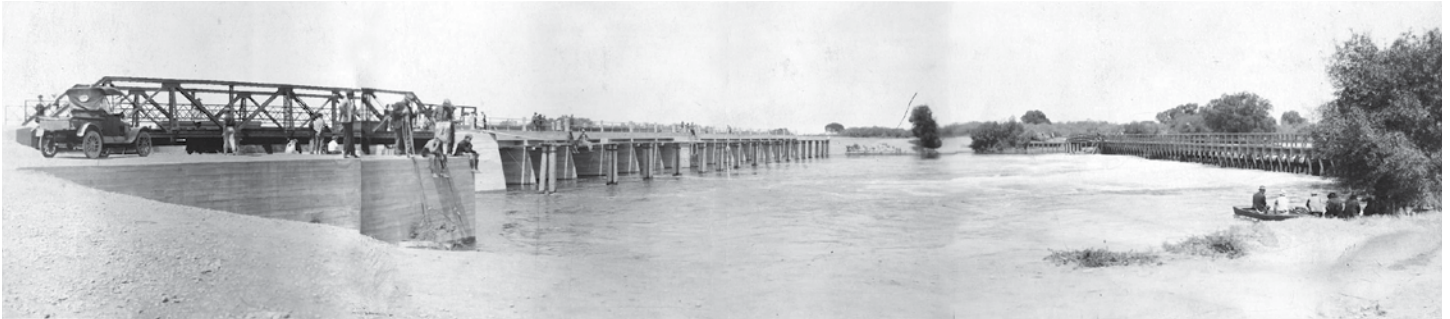
THIS HISTORICAL PHOTO TAKEN OF THE MENDOTA DAM IN 1919 SHOWS THE ORIGINAL STRUCTURE, AT RIGHT, JUST BEFORE IT WAS REMOVED, AND THE CURRENT DAM JUST AFTER IT WAS CONSTRUCTED. THE DISTRICT IS PLANNING SIGNIFICANT RENOVATIONS TO THE DAM THIS YEAR.
